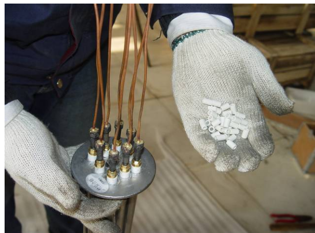
put the ceramic bead to the live line
