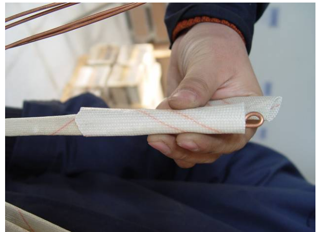
Protect the live line joint with \varnothing 16 wax duct
