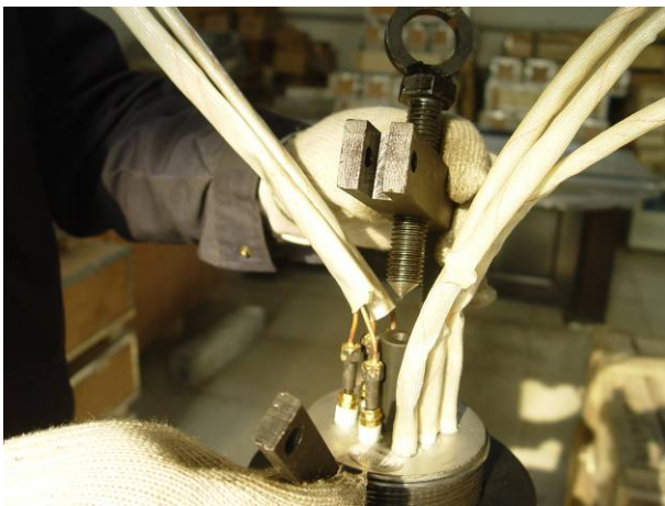
Fix the beam and the jackscrew
