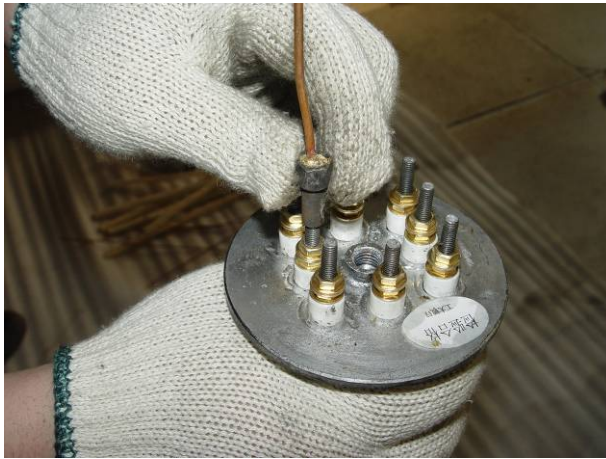
Put the wiring terminal
