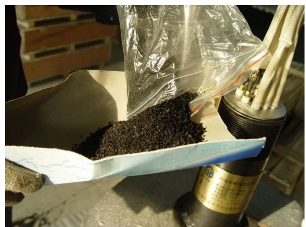
pull up the element a little and add carbon
