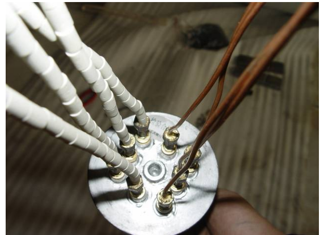
connect the heating core to control cabinet
