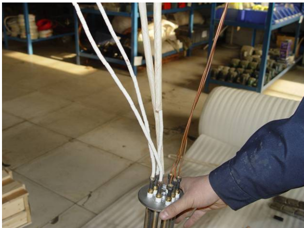
Protect the live line with \varnothing 12 wax duct
